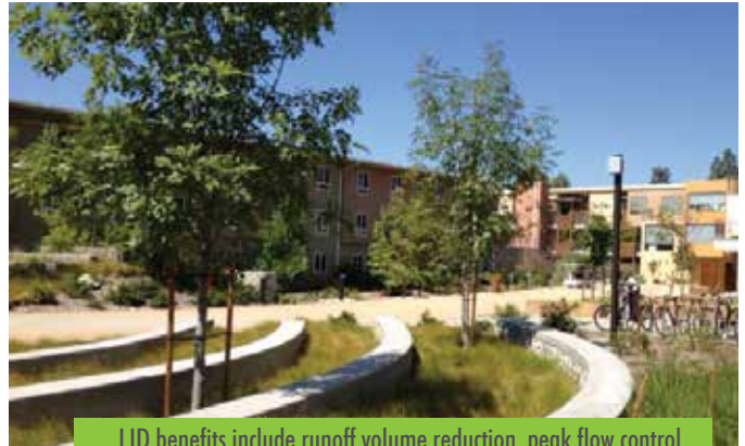
LID benefits include runoff volume reduction, peak flow control, ground water recharge, and water quality improvement.
